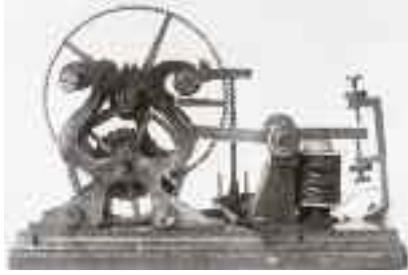
Morse's telegraph, which sent its first message on May 24, 1844
